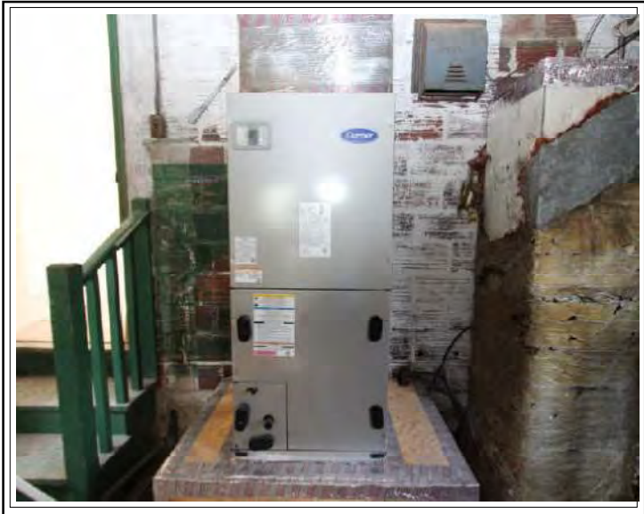
Carrier Air Handler - Dated May 2021 No Compressor Installed
