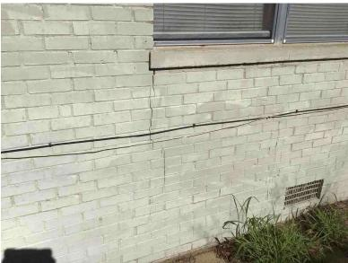
Apparent possible structural crack on home... Required to be inspected by qualified licensed structural engineer and remediation as per their report and recommendation
