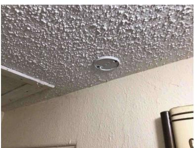
Smoke detectors missing and must be installed
