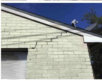
Apparent possible structural crack on home... Required to be inspected by qualified licensed structural engineer and remediation as per their report and recommendation
